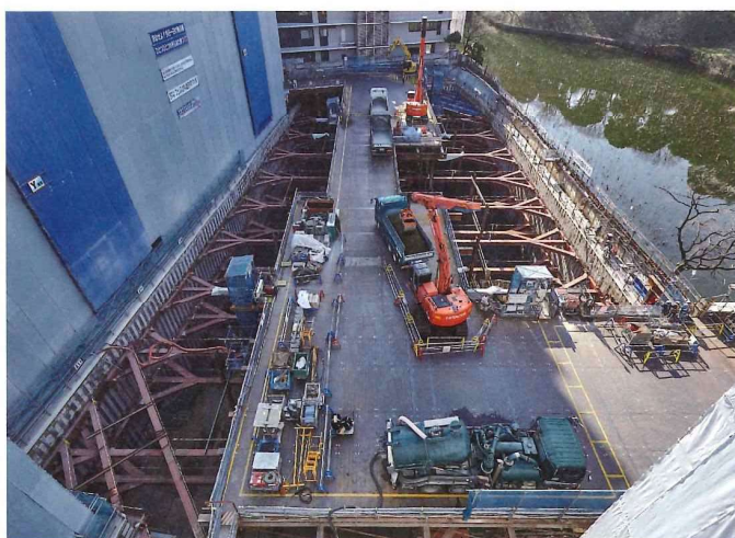
3次掘削施工状況(全域)。 | The third excavation construction (whole area).
