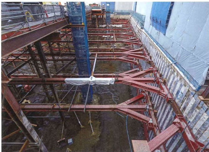
3次掘削施工状況。 | The third excavation work.
